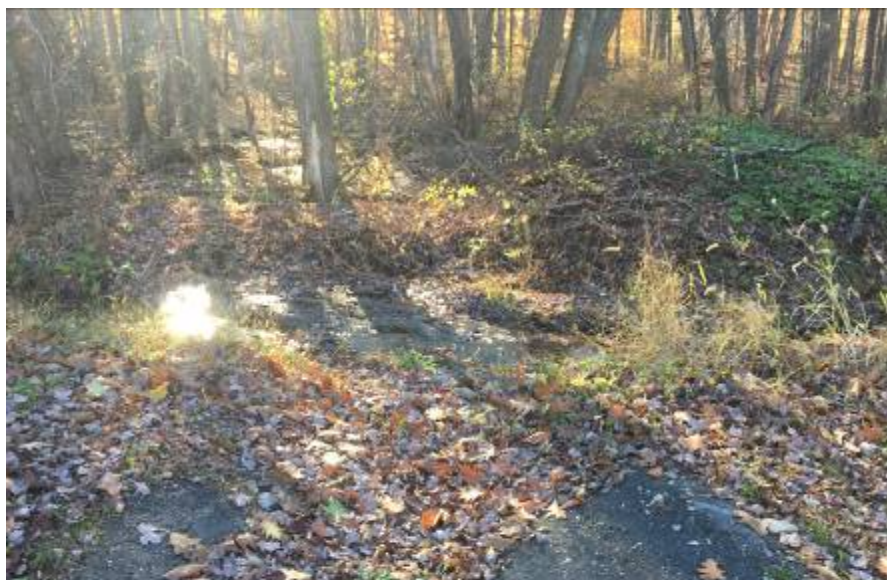
Asphalt sluiceway draining stormwater into man-made ditch at entrance to parcel
