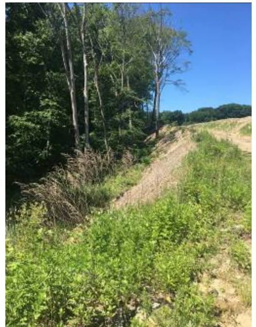
Cleared embankment could be stabilized with native vegetation to protect the nearby stream
