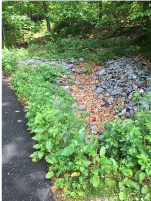
Rip-rap preventing erosion, a practice that can be used throughout Trumbull
