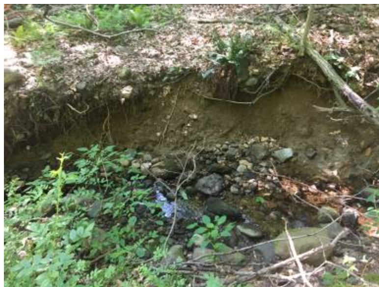
Storm water erosion from culverts
