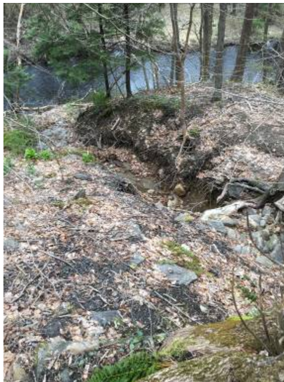
2. Eroded drainage ditch flowing into River 1.32 miles north of entrance
