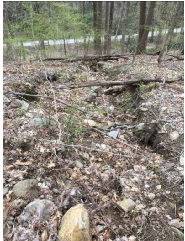
5. Eroded drainage ditch below hillside along Lakewood Drive
