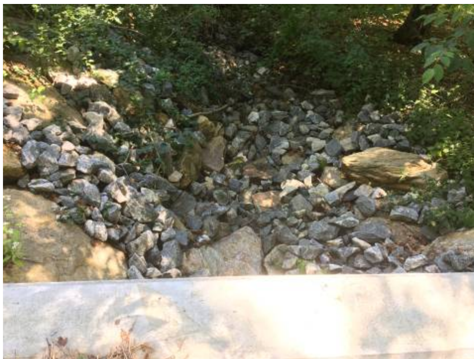
Newer culvert with adequate amounts of rip-rap at Towerview Drive
